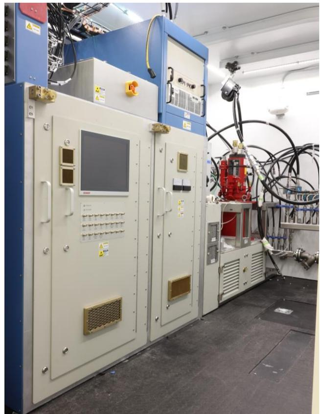
**Figure 2 – X-Band TWT transmitter configuration installed. The TWT is on the right (red).**
