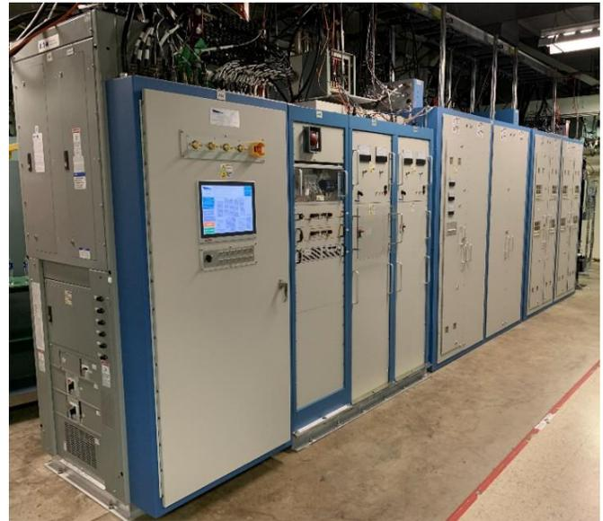
**Figure 2. COBRA DANE radar transmitter group replacement with (left to right) Controls Cabinet, Auxiliary Rack, HVPS 1 & 2, Capacitor Bank Cabinets (two) and Modulator Cabinet.**
