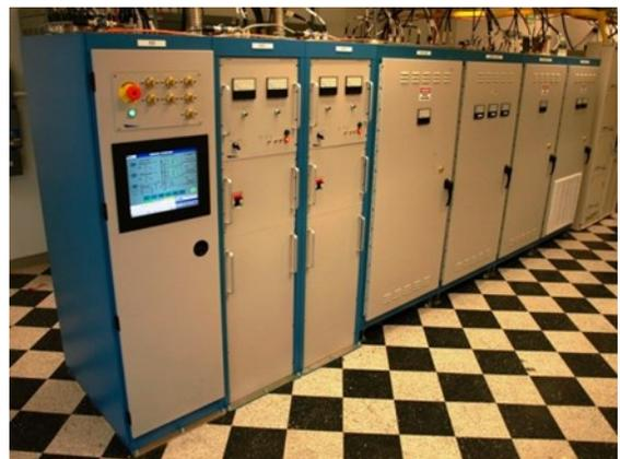
Figure 1. Installed Shore Power Feed Equipment.
