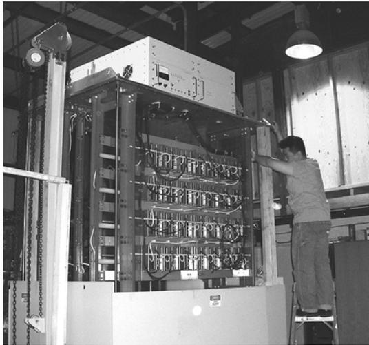
Figure 3. Installation of Sondrestrom modulator (150 kV, 300 A). The modulator's high voltage components are suspended from the tank lid. The assembly can be lifted out of the tank using an internal chain lift or an overhead crane.
