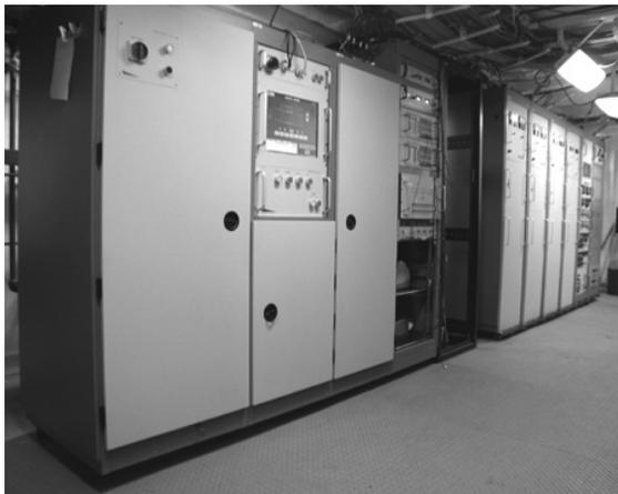
Figure 2. Cobra Judy X-band DC power supplies and controls installed on-board the USNS Observation Island.
