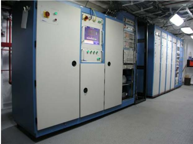
Figure 3. Cobra Judy X-band DC power supplies and controls installed on-board the USNS Observation Island.
