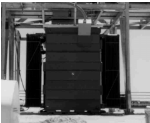
Figure 4: 2 MW Transformer
