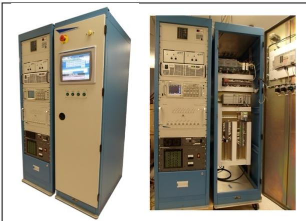
Figure 6. Controls racks for the 2 MW klystron transmitter.
