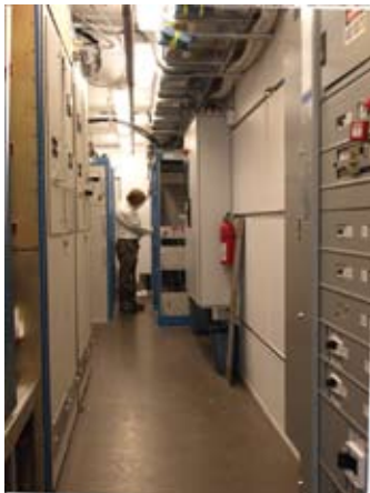
Shelter interior showing typical arrangement of transmitter components. DTI recently delivered X-band and S-band solid state, transportable radar transmitters configured in standard 45 foot, weatherproof ISO shelters to the U.S. Government.
