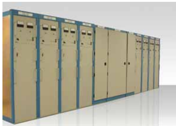
Cobra Judy S-Band transmitter power supplies.
